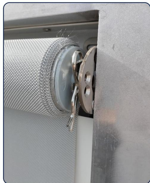
Insert the R-clip locking pin in place
