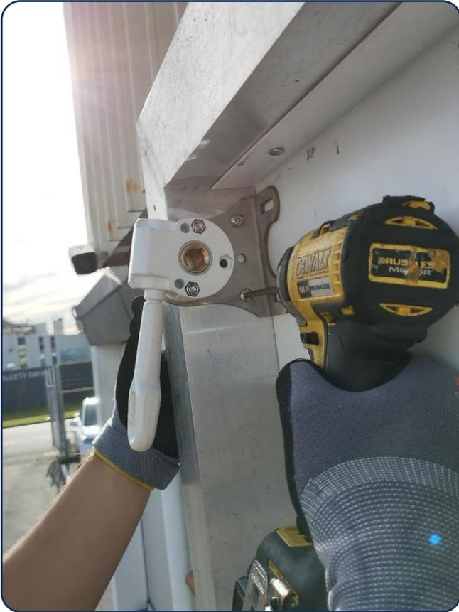
Screwing in the Gearbox bracket – Take note: the angle of the crank
