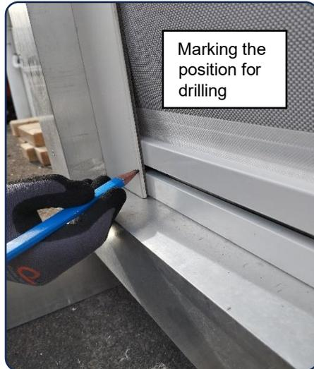
Marking the position for drilling
