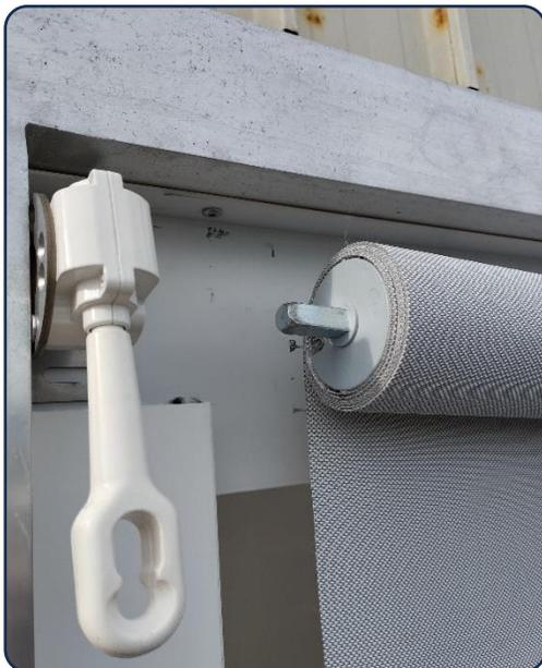
Inserting the square end into the gearbox
